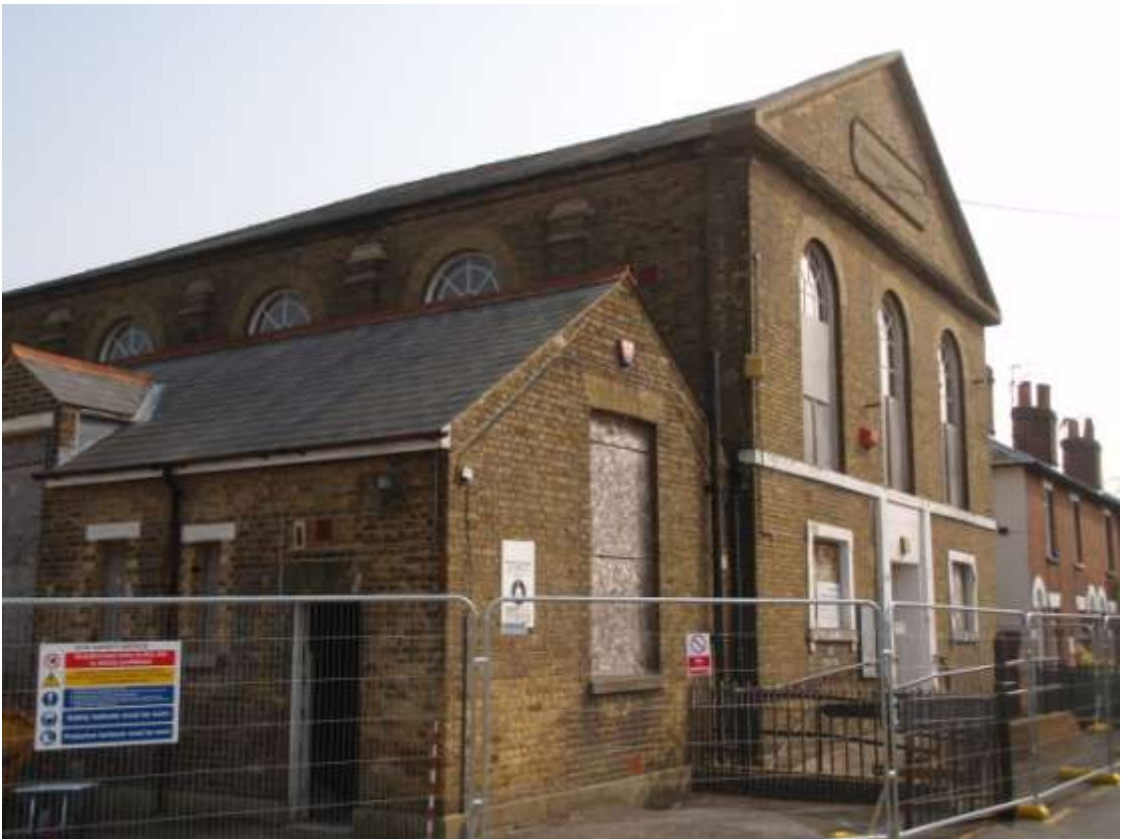
Plate 2. View of building (looking SE)
