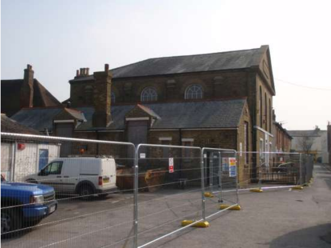
Plate 3. View of building (looking SE)
