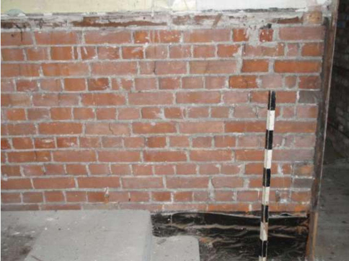
Plate 7. View of internal brick detail
