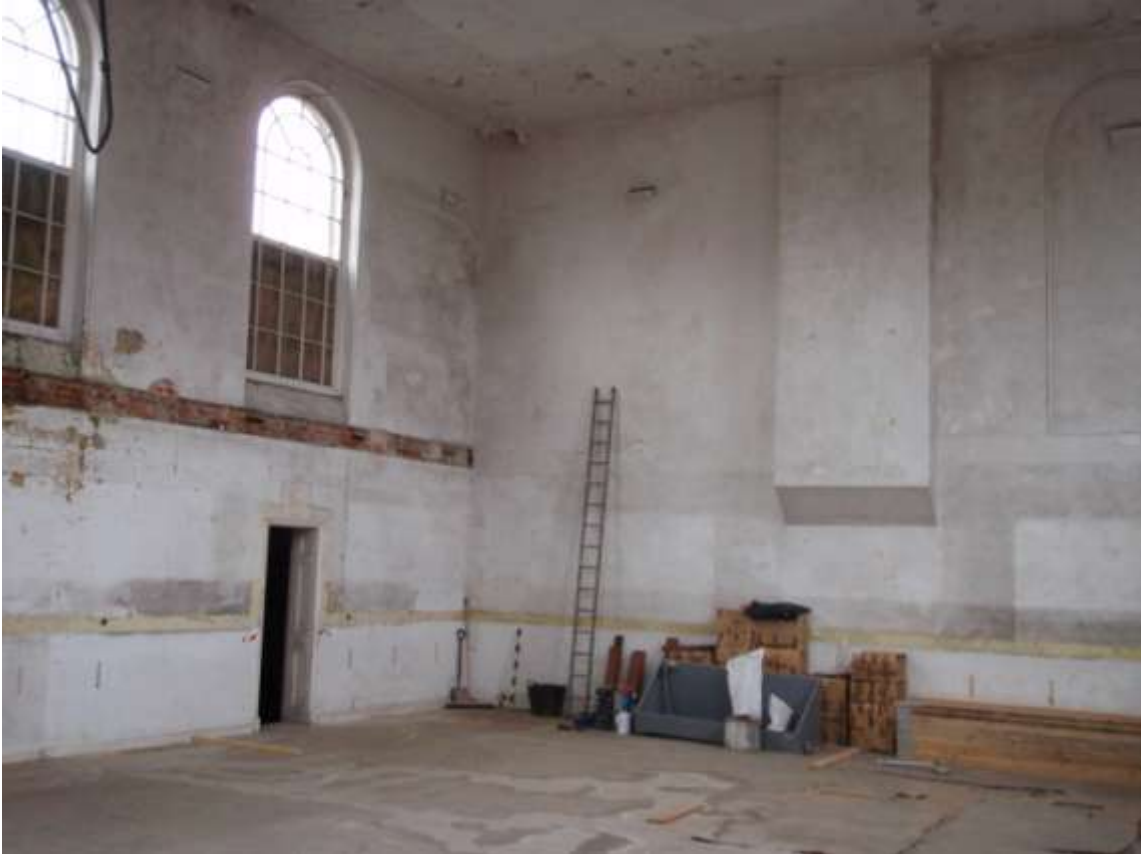
Plate 9. View of interior (looking SW)
