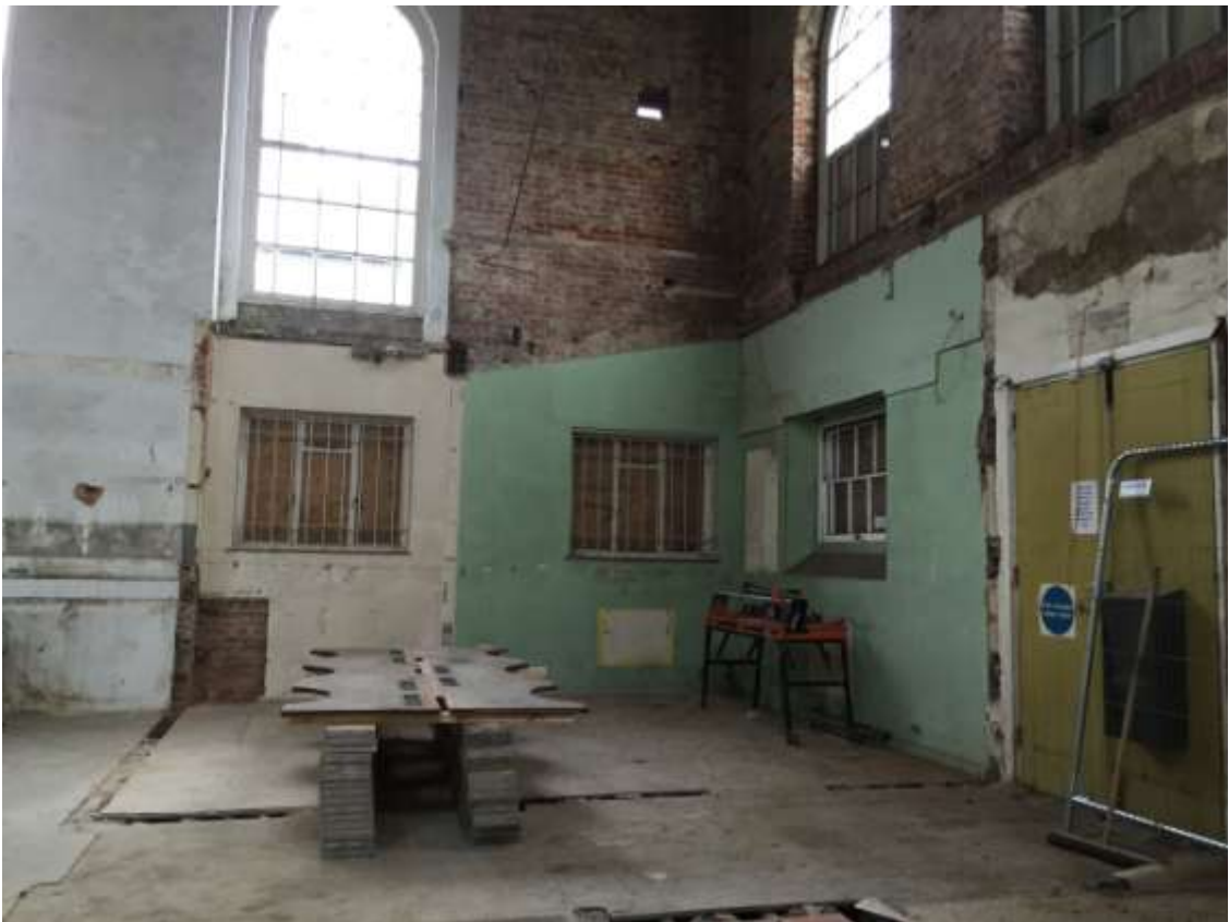
Plate 6. View of interior (looking SE)
