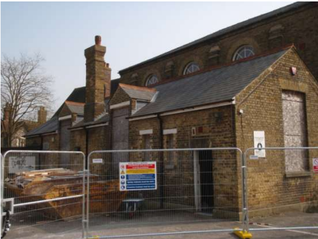
Plate 4. View of building (looking SE)
